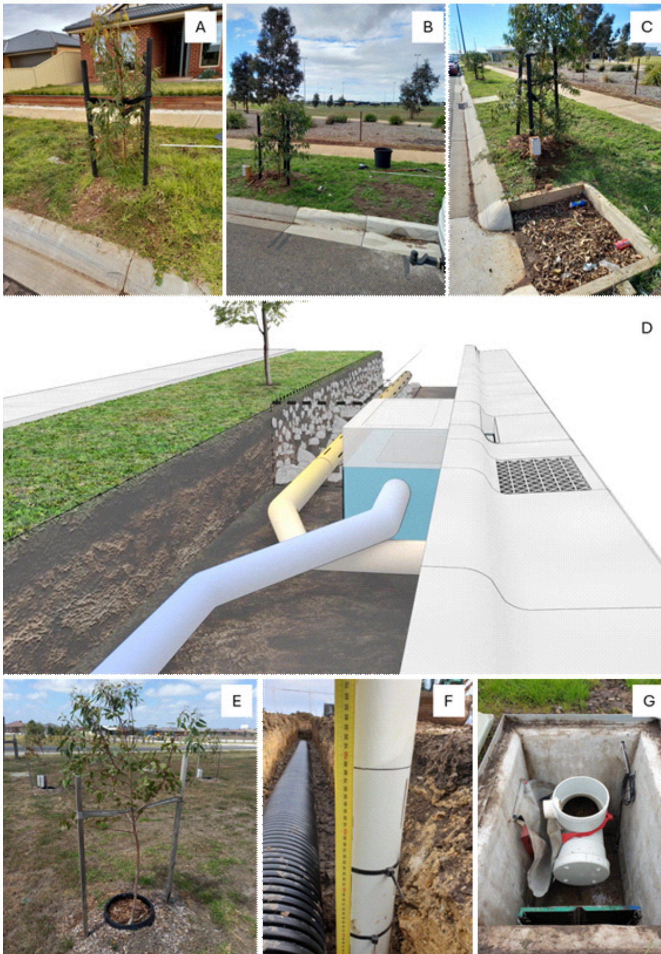
Figure 1: Melton field experiment where infiltration trenches receive stormwater from A) private roofs, B) lintel inlets and C) kerb cuts. D) shows a “big storage” concept designed for a typical suburban nature strip and E-G) show this design as tested in Cardinia Shire where E) trees are planted alongside F) an infiltration trench filled with structural soil with G) an internal water storage created by a downstream pit riser.
